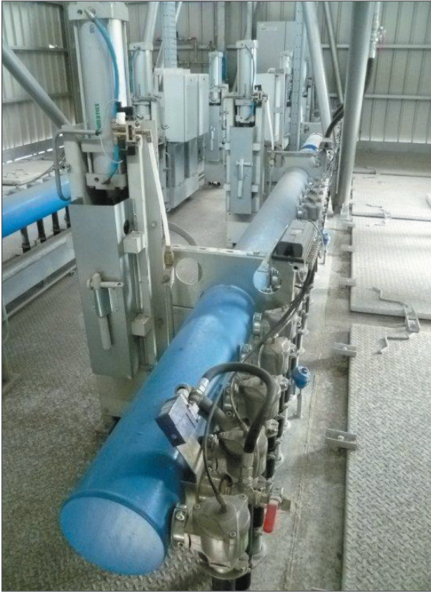
Conditioning with reverse-jet method, spool valve with patented quick connection (clamp) and Cylinder-Valve combination for damper control.
